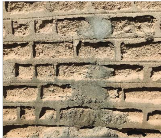
Figure 5: Sea-sand bricks with cement mortar in the buildings of the 1960s
