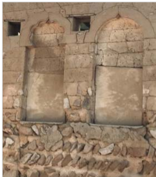
Figure 3: Coral stone walls in buildings of the 1950s
